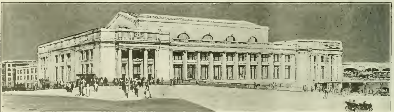
NEW UNION STATION, ST. PAUL, MINN., UNDER CONSTRUCTION
